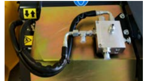
Oil Flow Control Available on all L/SL buckets to control oil flow speeds.
